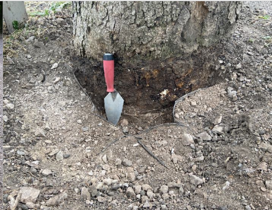
IMAGE 5: The excavated path surface to the south side of the trunk.
